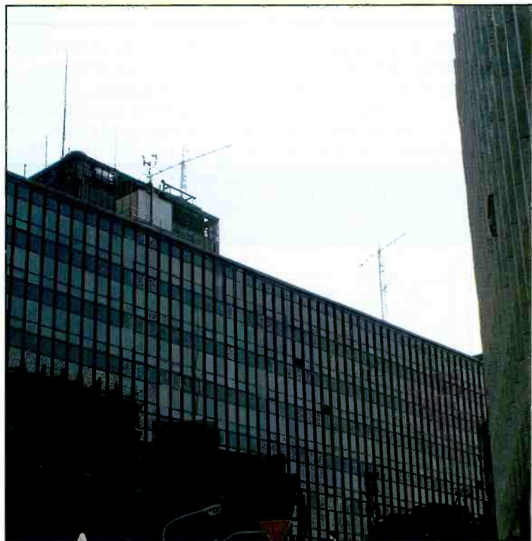
The Kyodo News building with two log periodic antennas seen on the roof.
